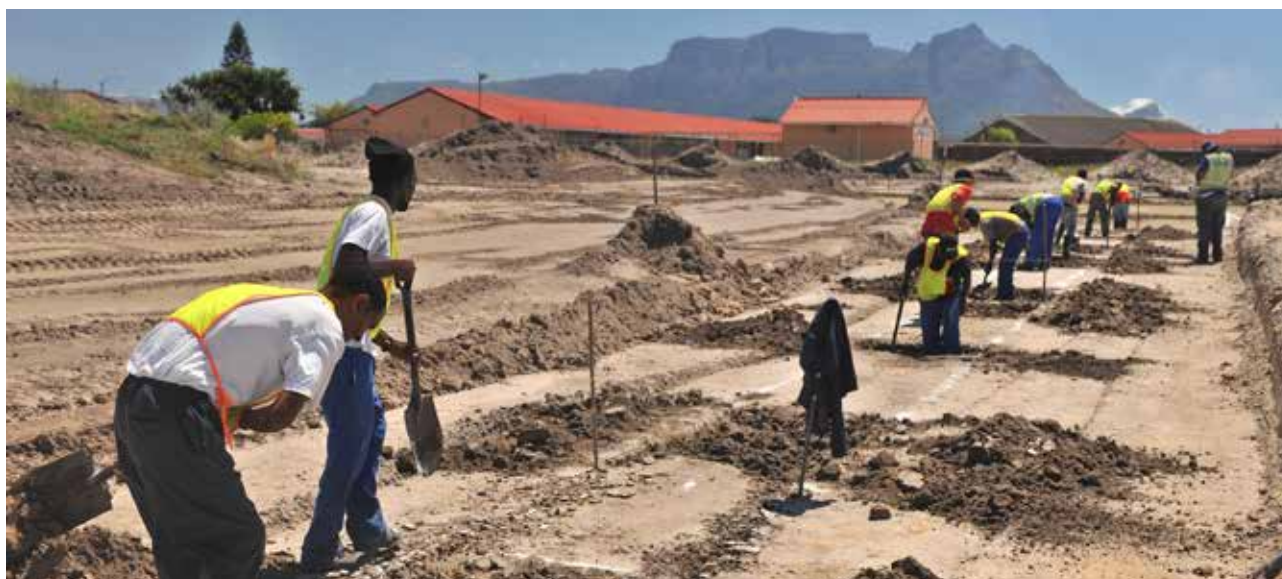
Preparation for a new housing development.
